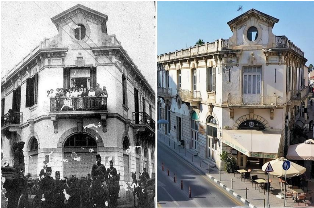
An old picture of the building (1917) and the most recent one (2019).
