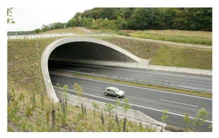
**Figure 28.** An overpass built near Žehuň (Central Bohemia region, Czech Republic) to allow wildlife crossing D1 motorway. Photo: I. Dostál (CDV).
