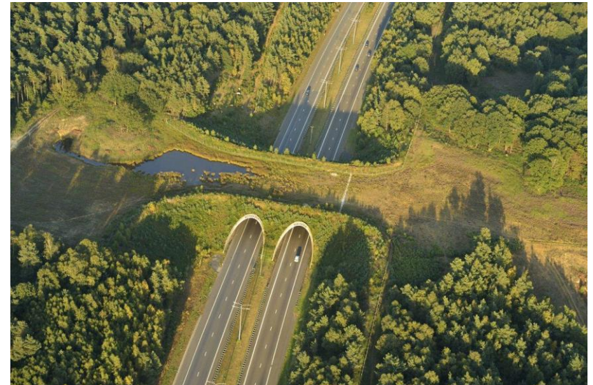
Wildlife overpass in Belgium.
