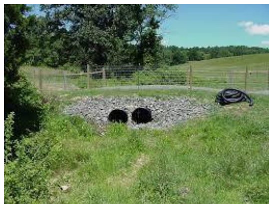
Figure 5. Culvert crossing. Source:
