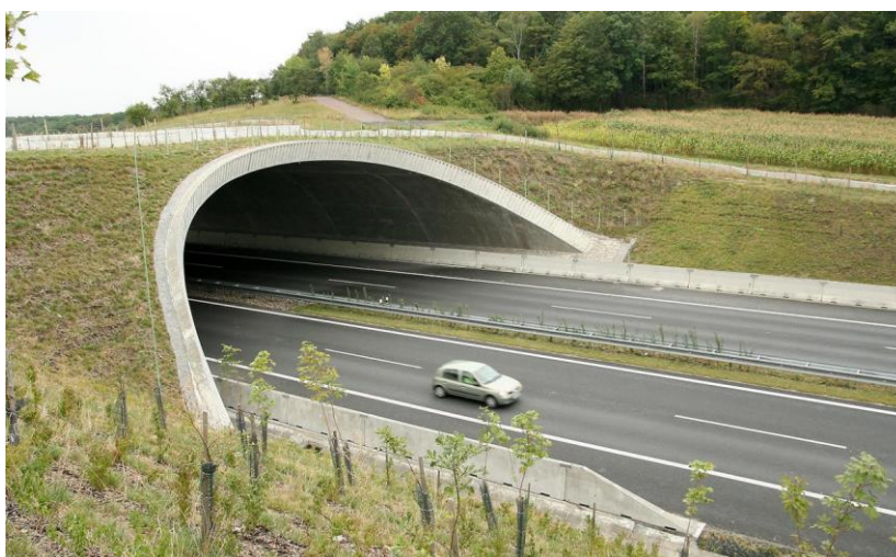
Figure 28. An overpass built near Žehuň (Central Bohemia region, Czech Republic) to allow wildlife crossing D1 motorway. Photo: I. Dostál (CDV).
