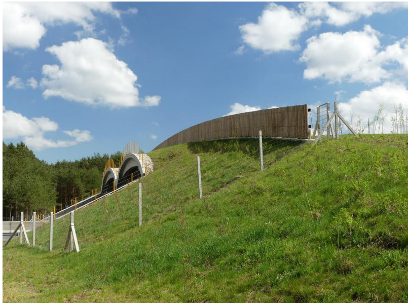
Figure 6. An overpass, accompanied by fencing, across D2 motorway near Bratislava, Slovakia. Note the wooden barrier on the top of the overpass to block view of animals when crossing. Photo: M. Králík (HBH).
