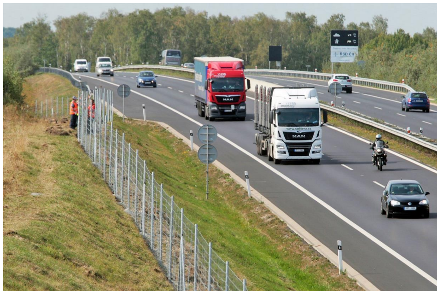
Figure 3. Fencing along roads is capable to block movement of large mammals. Photo: Václav Šlauf, MAFRA, Czech Republic.
